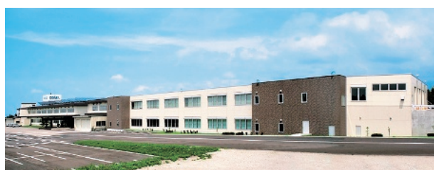
Company building: Tateyama Factory
